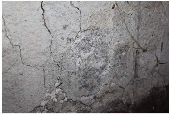
(c) map cracking
