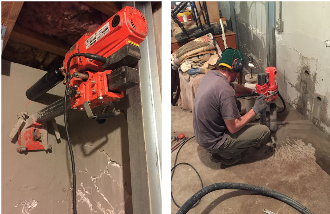
Fig. 4.1 Coring process carried out by a third party contractor
