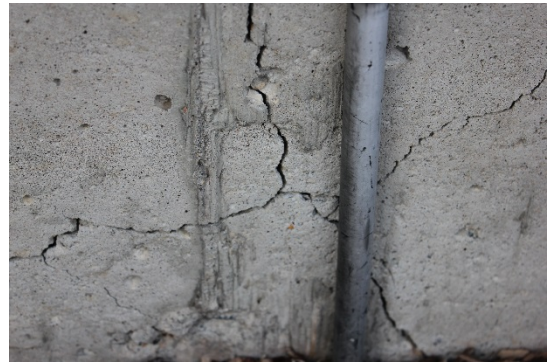
(b) map cracking
