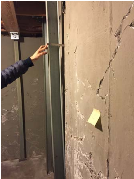
e) significant deformation of the concrete foundation wall
