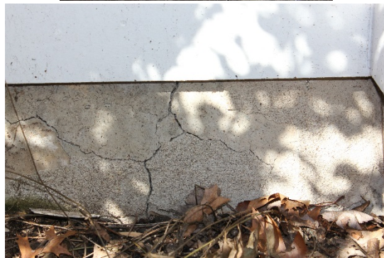
(b) map cracking
