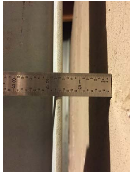
e) significant deformation of the concrete foundation wall
