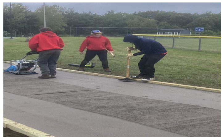
Leveling out the top layer.
