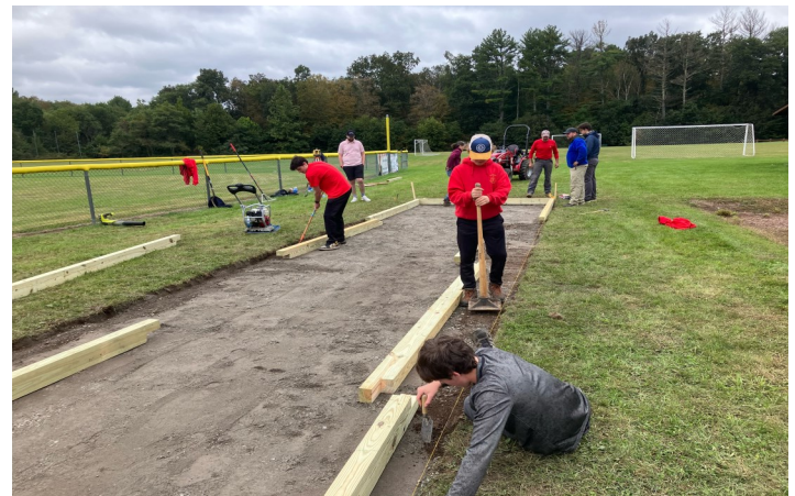
Installing the border of the court.
